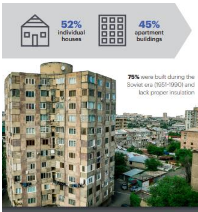
Fig. 3. 75% building were built during the Soviet era (1951-1990) and lack proper insulation (Energy-efficient buildings in Armenia: a roadmap, IEA, EU4Energy, 2020)
